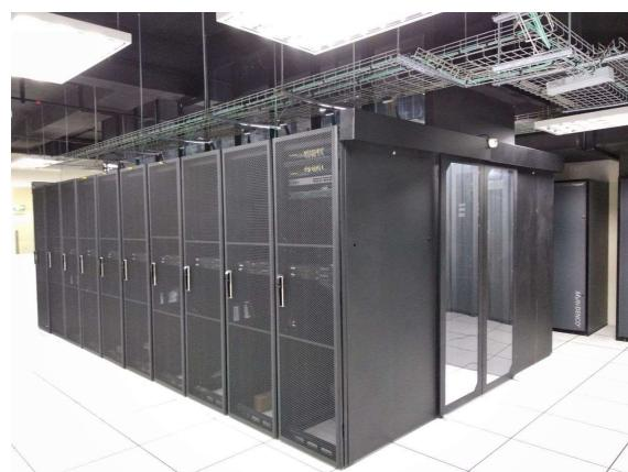
CKD Containment Frame, Sliding Auto-Close Aisle End Door, Swing Auto-Close Aisle End Door, Rack-Space Blanking Acrylic Panel, Fire Triggered Down-Swing Top Acrylic Panel, 1.5mm CR Plate, 3.0mm Acrylic Sheet
